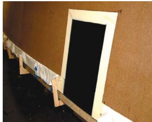
Nomex® honeycomb fit around the chain plate on a 65' hull.
